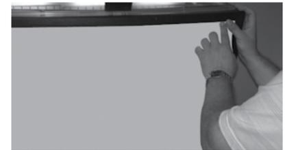
5. Finish installing the graphic by feeding the top right corner of the graphic into place.
