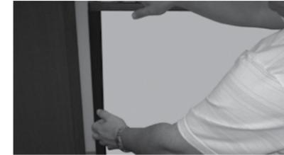
2. Feed the top of the graphic into the top left graphic channel.
