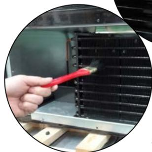
4 Using plastic bristle brush, carefully clean the coil being aware that coils can bend or be damaged if too much force is used - shown left.
