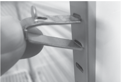
Securely insert shelf clips into pilasters
